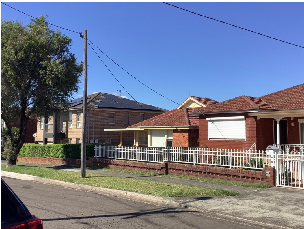
Figure 8: view of opposite neighbouring properties to the North
